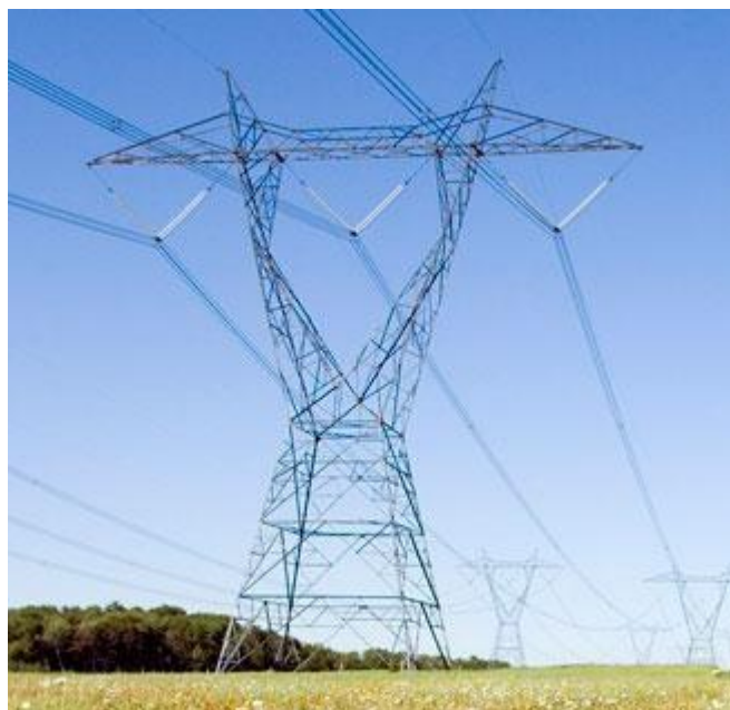
Figure I.8: pylône nape.
